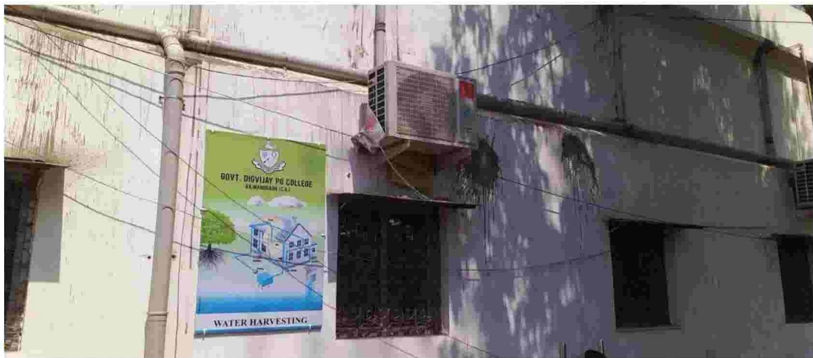
Fig: The installation of Rain water Harvesting System is adding more to the already sufficient ground water level.
